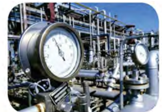
Condensate line pressure gauge AFTER GEM Traps (90 PSIG)
