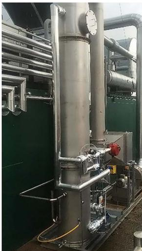
Creamery customer runs a 600KW electrical output Combined Heating and Power (CHP) plant, 24 hours a day. The CHP, also known as CoGeneration (CoGen), is used to generate electricity for supply to the grid. Thermal Energy International (TEI) identified that significant savings could be achieved by utilising the waste heat from the waste gasses and the engine cooling jacket.
