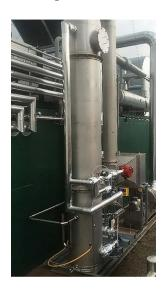
Creamery customer runs a 600KW electrical output Combined Heating and Power (CHP) plant, 24 hours a day. The CHP, also known as CoGeneration (CoGen), is used to generate electricity for supply to the grid. Thermal Energy International (TEI) identified that significant savings could be achieved by utilising the waste heat from the waste gasses and the engine cooling jacket.
